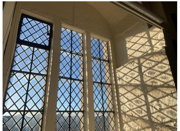
Newly renovated ringing room window
